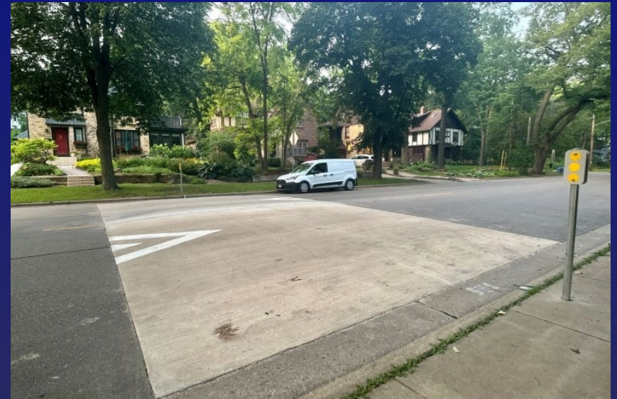
Concrete Speed Table (Madison, WI).
