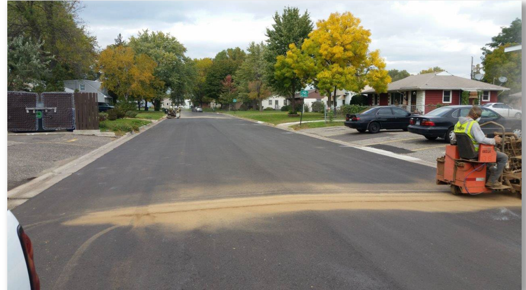
Pavement saw & seal
