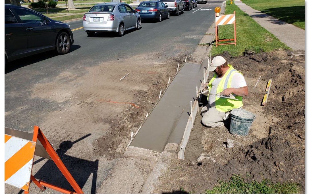
Finishing spot curb & gutter replacement
